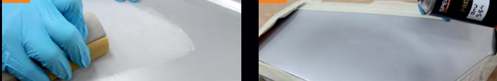
6. Mask the adjacent surface and apply the ACRYLIC PRIMER on the area of repair.
